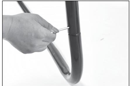
2. Assembly legs (C) to the leg extender bar (B) using the little screws (D) and Allen key (E).
